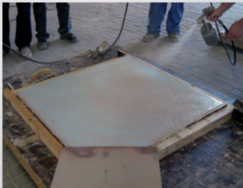
apply the retarder on fresh concrete
