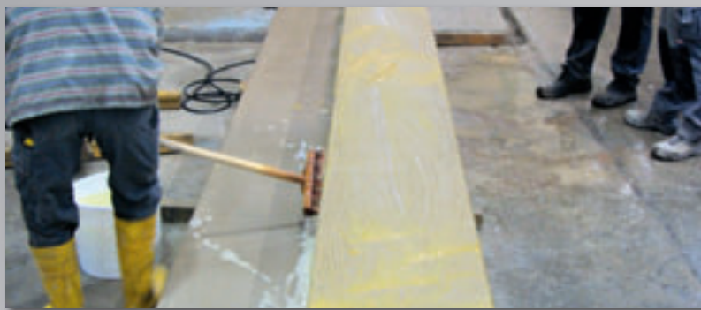
apply the cemgel with a soft broom
